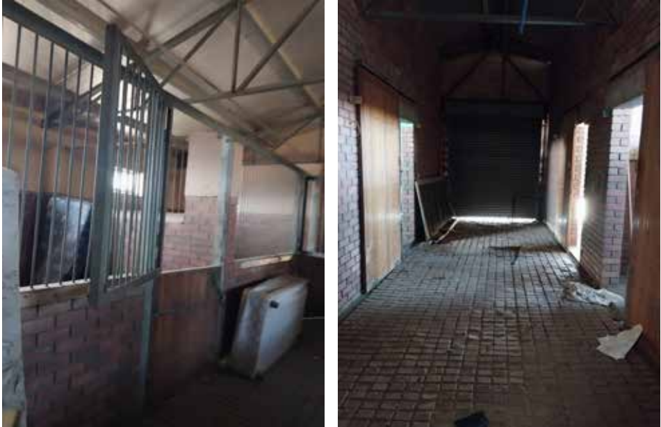
Figures 1 and 2: Building condition before renovation
