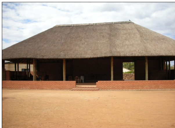
Figure 5: A low-rise masonry wall is used to define the open area with a thatched structure for the elders in a modern-day Kgotla (Source: Moumakwa, 2010, pp. [i], 52)
