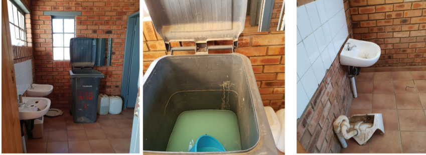
Figure 1: Unsanitary conditions of toilets at School A. The black bin is used to store water with chemicals used to flush the toilets throughout the day. (Photos: Kyle Odgers, 2018)
